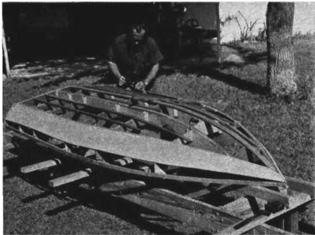
**SPLIT** keel along thickest part so it will bend easily to take the shape at front.
