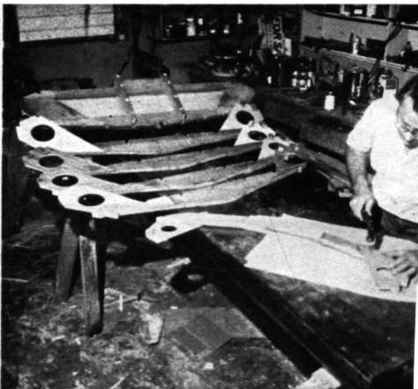
**CUT ribs and transom from 1-in. stock and use cardboard template to get shape. Note the use of glue blocks at the ends of ribs.**
