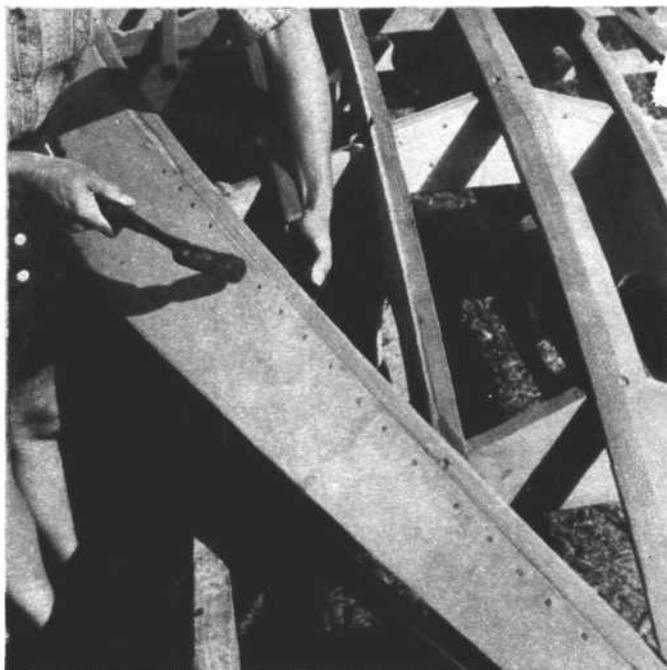
**BOTTOM** planking goes on with glue and nails. Use backing block for nailing. Note reinforcing blocks at rib/girder juncture.
