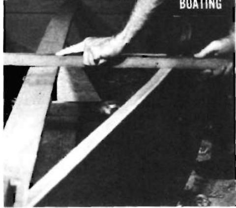
The final job before the bottom goes on is that of checking the planking job with a "fairing" stick, which measures flatness for installing the bottom.
