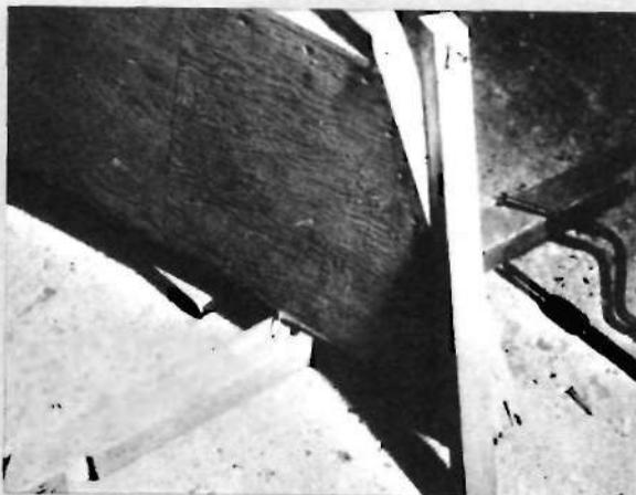
The final touch for the nose is the outer stem. It will be planed to a taper after screwed into place.
