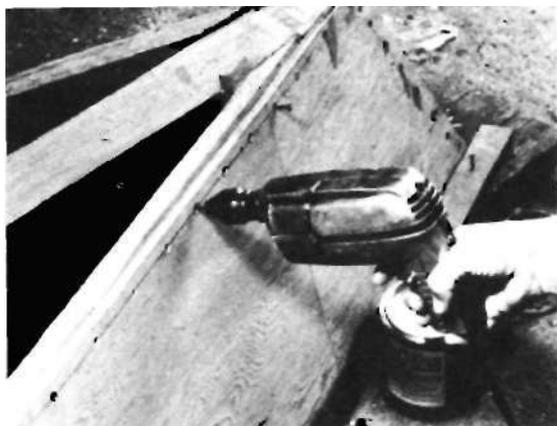
Chine goes into notch cut for it in transom. Note the two screws joining the inner keel to transom.
