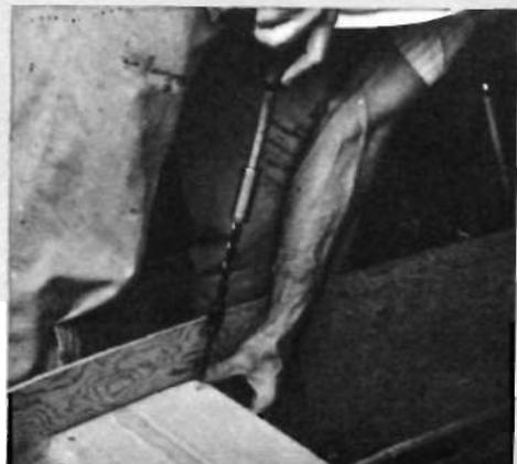
Sheer rail is rabbeted to mount atop side panels, serving as frame plus rib rail. Screw holds batten.
