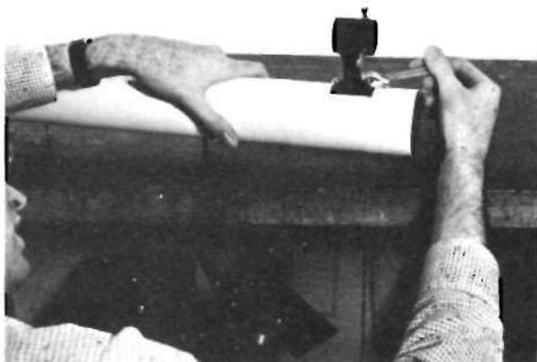
Before going on, a word of caution: NEVER DROP lenses into the casing. Follow photo instructions here. Next, fasten finder-mounting on scope-tube.
