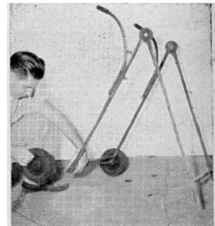
**Supporting frame.** Two identical sides with handles are welded over layout drawn with chalk on cellar floor. Sides are braced to stand vertically and cross members added. Short lengths of  $7/16$ " rod for axles are welded into lower cross member at rear.
